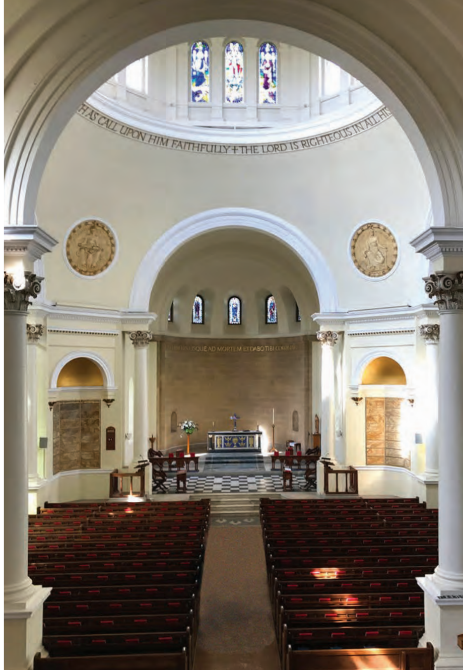
4. Right: In the inter-war period, the High Victorian Chapel and its decoration was considered devoid of charm. Demolition was inconceivable, so in the mid-1930s Baker was asked what could be done. Internally, he cleverly inserted an inner dome, complete with inscriptions, that transformed the character of the space. Externally, he replaced the original, windowless apse with a larger apse in the same brick as the newly-completed Memorial Hall (see photo on page 7). The apse has the Baker trademark of five small high-level windows.
