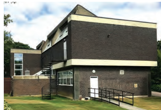
Above: The Art School by Porri & Foyle (1965) was a bold break with Haileybury's architectural precedents. It is in the 'brutalist' style of the 1960s. The materials – dark engineering brick and concrete – are tough and are used in an uncompromising, almost aggressive, way. The Art School was, and still is, praised for its practicality.
